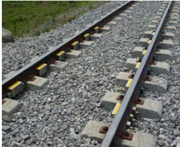
Figure 2: Picture of a wheel impact load detector installation, where the individual measurement devices are shown in yellow.
